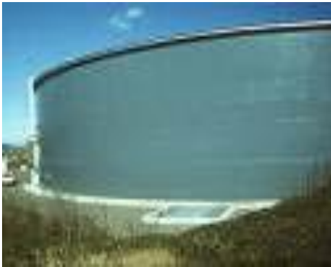
Welded Steel Tank
