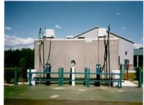
Encased in concrete
