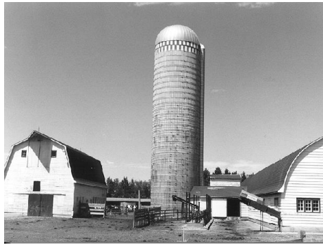
Concrete Poured Silo
